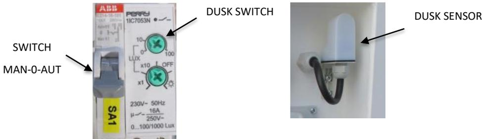
The electric panel includes a dusk relay and its relative dusk sensor, controlled by a switch. When the switch is on MAN, the dusk relay is bypassed and the floodlights operation is according to the position of the relative switches.
