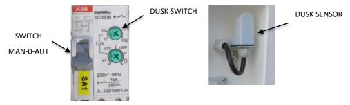
The electric panel includes a dusk relay and its relative dusk sensor, controlled by a switch. When the switch in on MAN, the dusk relay is bypassed and the floodlights operation is according to the position of the relative switches.
